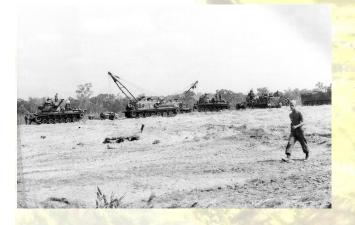
We were near Cambodia, repairing broken tanks on an isolated Fire Support Base. The tank repair vehicles have their booms raised to pull the engines out of the tanks. The new engines were flown in by a Sikorsky Sky Crane.
